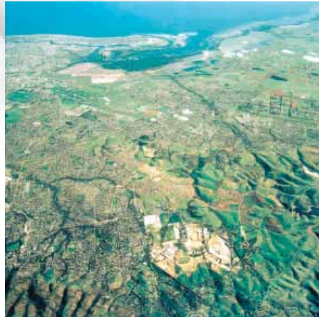
Above: Adelaide is one of the world's lowest density cities but the city's urban sprawl must be curtailed if Adelaide is to become a sustainable and green city. Source: Planning SA
